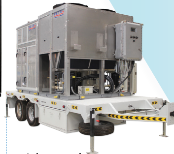
► Stainless Steel Explosion Proof Mobile Package Unit for Oil and Gas Projects
